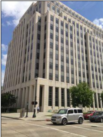
Galvez Building Baton Rouge, LA
